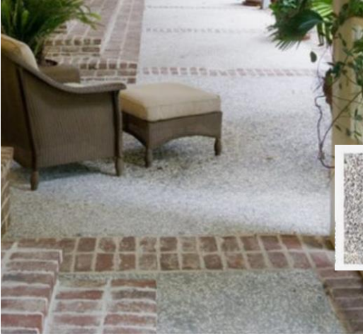
Terrace / Patio: Brick-edge with exposed aggregate in center Color: Red/Terracotta to match house brick
