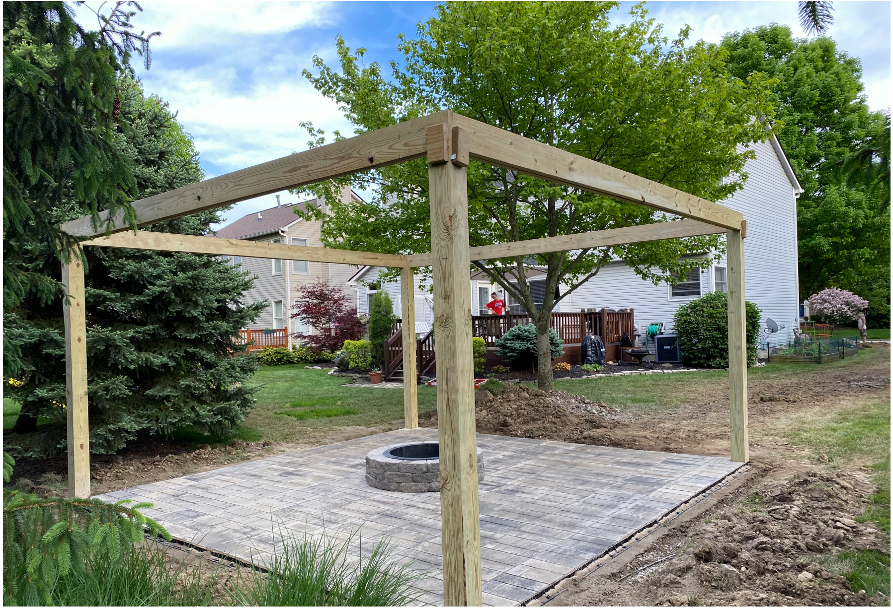
After: From NW corner of property facing house.
