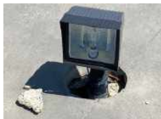
Current Conditions 5 Lighting exposed and deep hole in concrete deck
