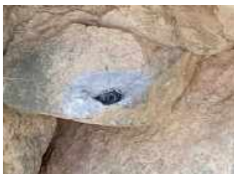
Current Conditions 4 Holes in concrete wall face
