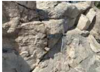
Current Conditions 2 missing chunks of concrete from wall face
