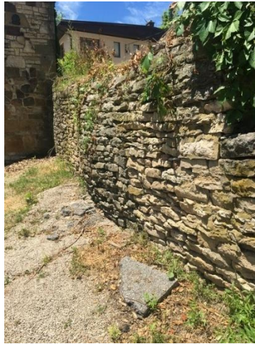
Retaining Wall Bulge at Mid-Height
