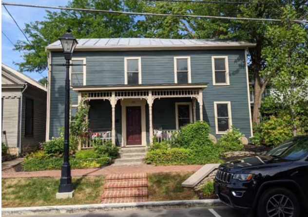
East elevation; existing structure
