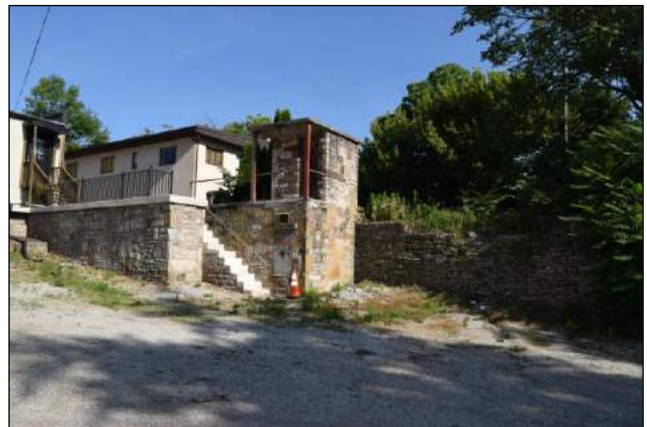
36-38 N High St, stone privy, looking northwest
